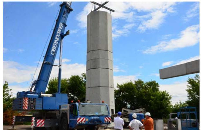
Fig. 1 Erected Prototype with an outer diameter of 4.15 m at the bottom and a total high amounting to 16,15 m
