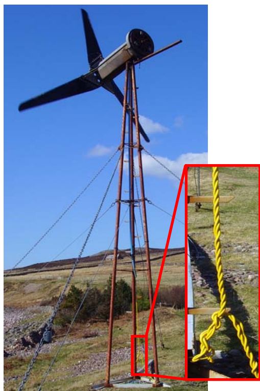
Figure 1: Cable twist on a small wind turbine without slip rings
