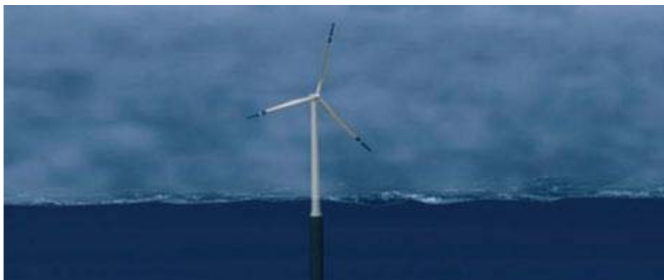
Figure 1: Floating wind turbine based on the Hywind concept [6].
