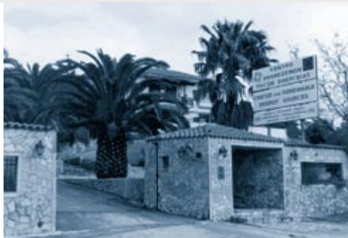
CRES, entrance to main facilities
