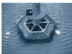
Scour protection at wind mill foundation
