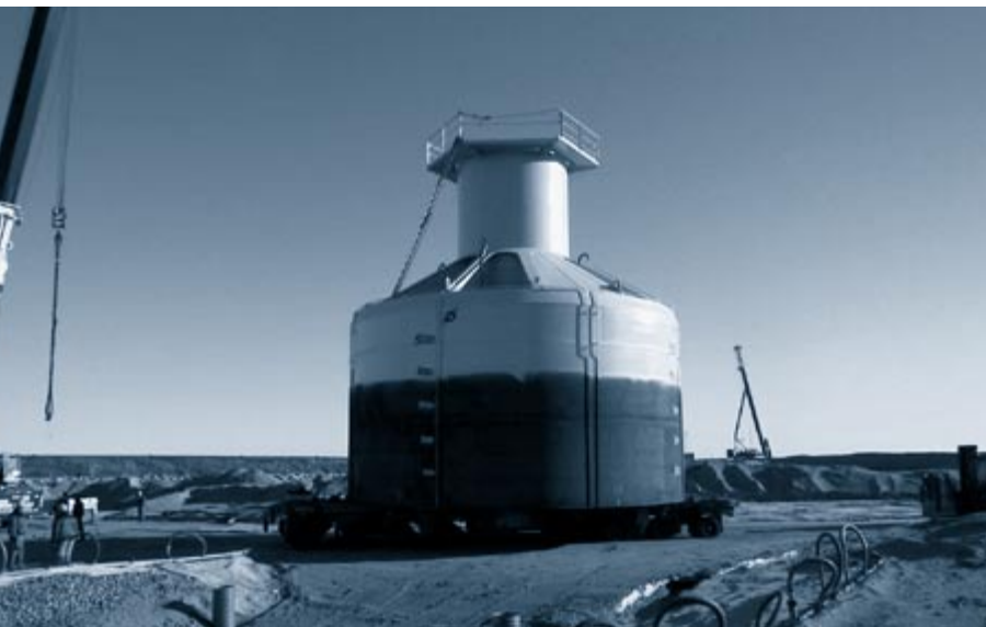
Foundation for off-shore wind turbine
